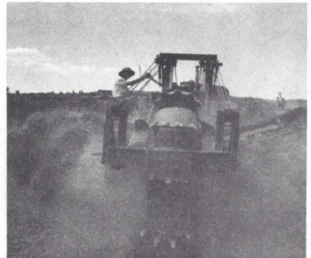
NEXT COMES THE TRENCHING FOR THE WATER MAINS.
