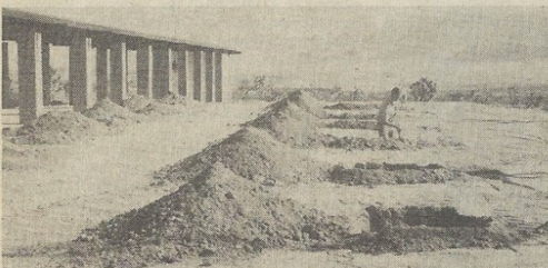
Ditches dug for wing footings.
