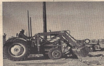
BACKFILLING OF WATER MAINS IS COMPLETE IN THE CAMPGROUND AREA. ELECTRIC LINES ARE NOW BEING INSTALLED FOR THE OVERNIGHTER SPACES.
